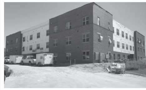
Libertad under construction. Located on SE 14th St. in Des Moines
